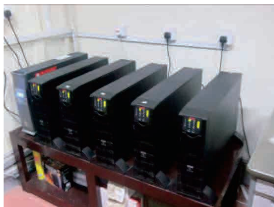
Figure 4-2-10. UPS units installed between power sources and ICT equipment
