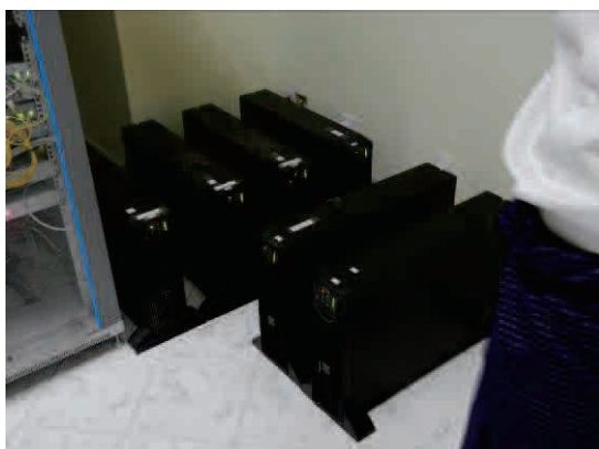
Figure 4-2-10. UPS units installed between power sources and ICT equipment
