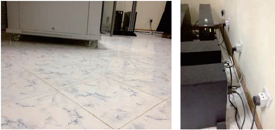
Figure 4-2-8. Racks not fixed to the floor (left-hand side) and ICT equipment placed directly on the floor (right-hand side)
