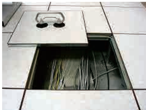
Ordinary data center floor (raised)
