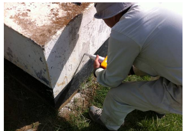
Rapid Sand Filter No.1 ⑨
