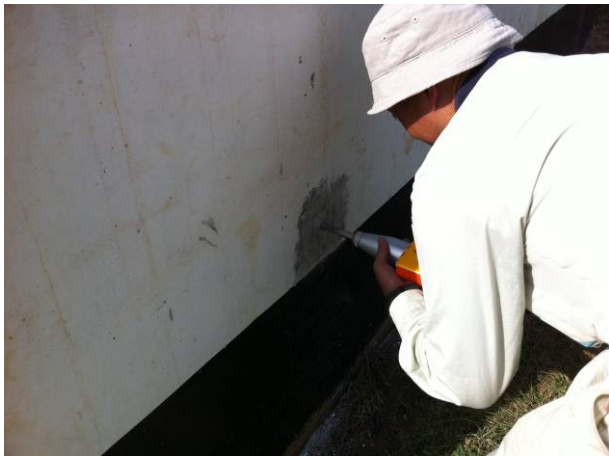
Rapid Sand Filter No.2 ⑮
