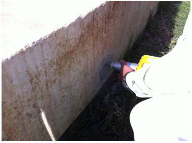
Sedimentation Tank No.2 ⑥
