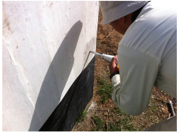
Rapid Sand Filter No.2 ⑭
