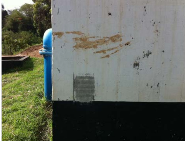
Sedimentation Tank No.1 ①
