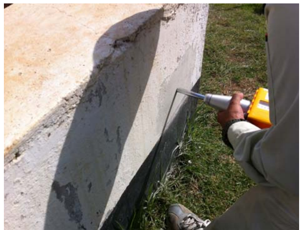
Sedimentation Tank No.1 ④
