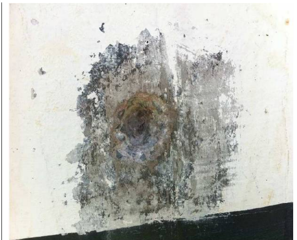
Rapid Sand Filter No.1 (BEFORE)
