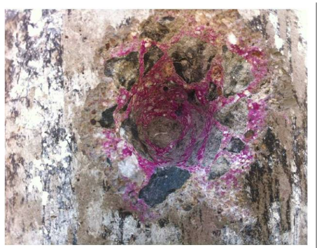
Rapid Sand Filter No.1 (AFTER)
