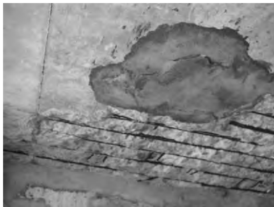
Block 1 Slab bet. Pile 1A& 2A-1
