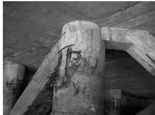
Block 1 Pile 2B-2
