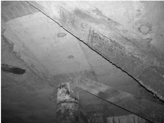
Block 3 Pile 61B
