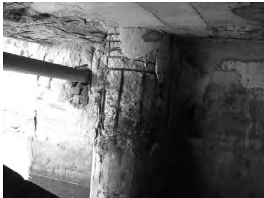
Block 1 Pile 1A
