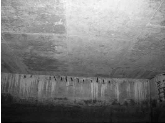
Block 2 Wall bet. Pile 18A & 19A
