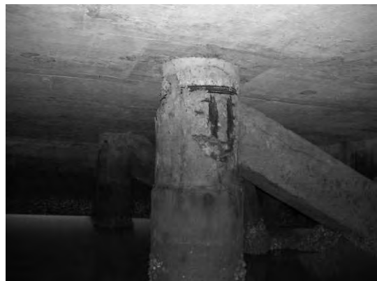
Block 3 Pile 61F
