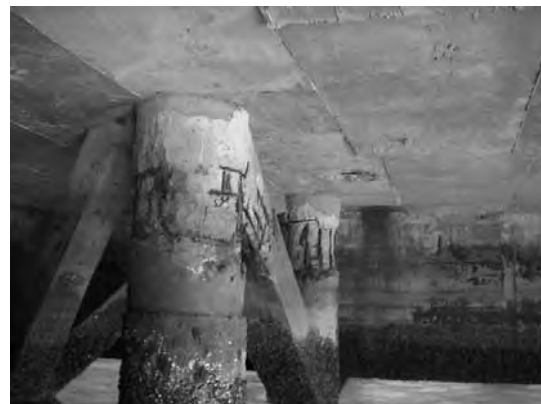
Block 1 Pile 2D-1
