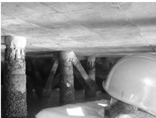
Block 1 Pile 2D-1
