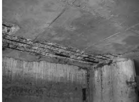
Block 1 Slab bet. Pile 1A& 2A-2
