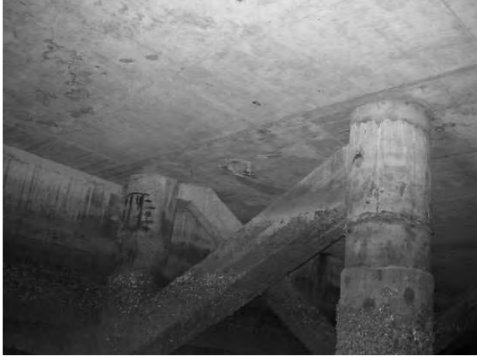
Block 3 Pile 60F ~ 60G-1
