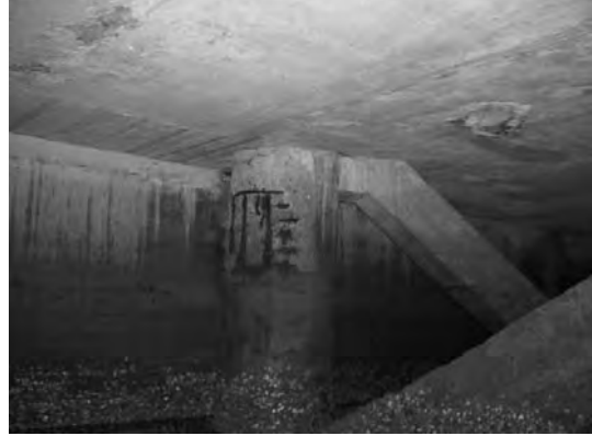
Block 3 Pile 60F ~ 60G-1
