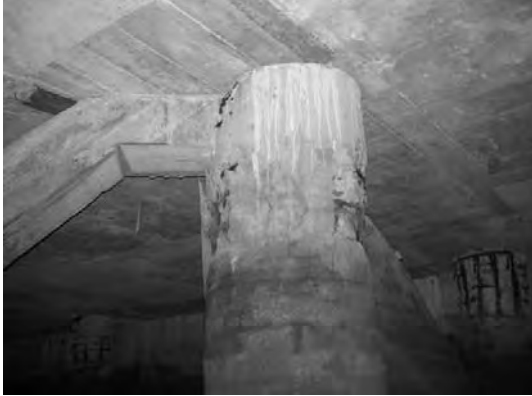
Block 2 Pile 20B
