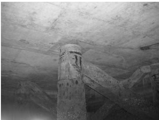
Block 3 Pile 61F
