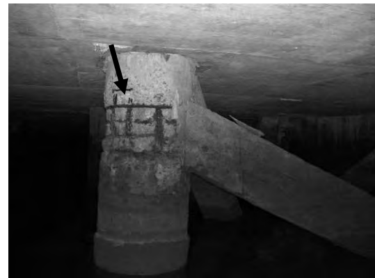
Block 2 Pile 39F
