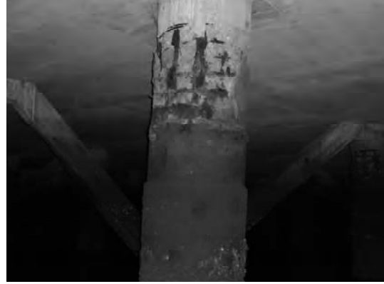
Block 3 Pile 50E-1
