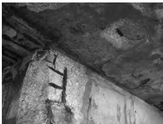
Wall and Slab nearby Pile 1C
