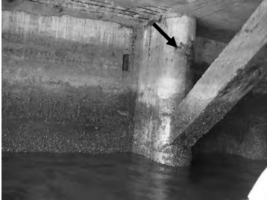
Block 1 Pile 2A
