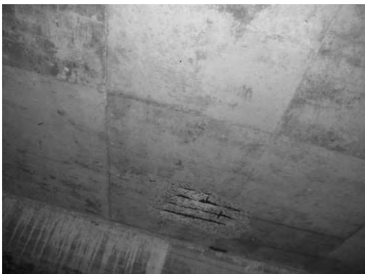
Block 2 Slab bet. Pile 20A & 21A
