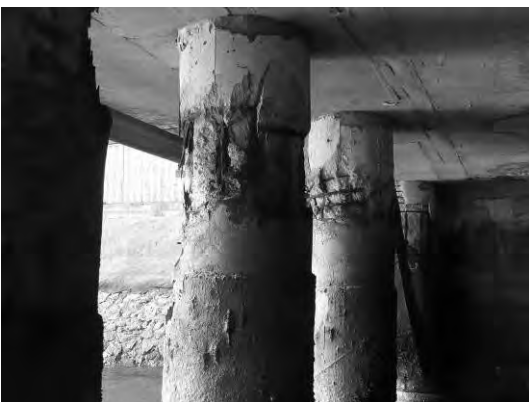
Block 1 Pile 1B & 1a
