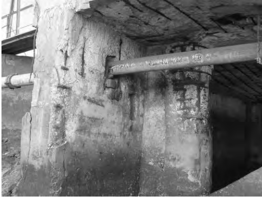
Block 1 Pile 1A and Wall
