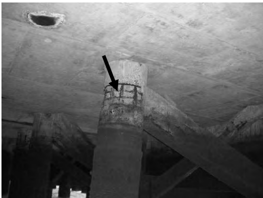
Block 2 Pile 39F
