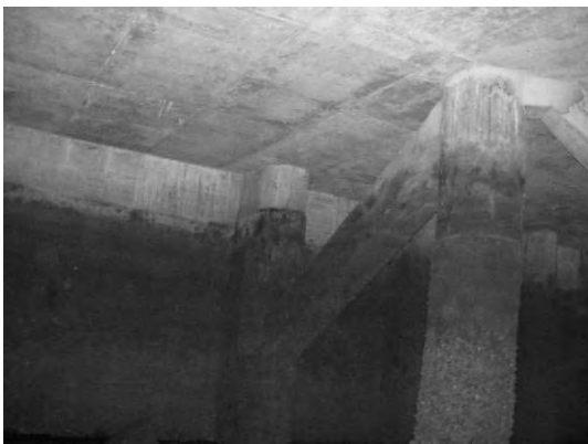
Block 2 Pile 39A ~ 39B
