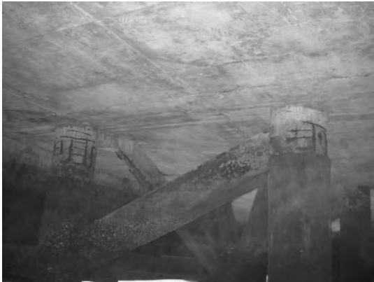
Pile 6B ~ Pile 6C
