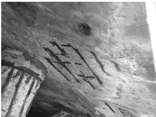
Slab nearby Pile 1B
