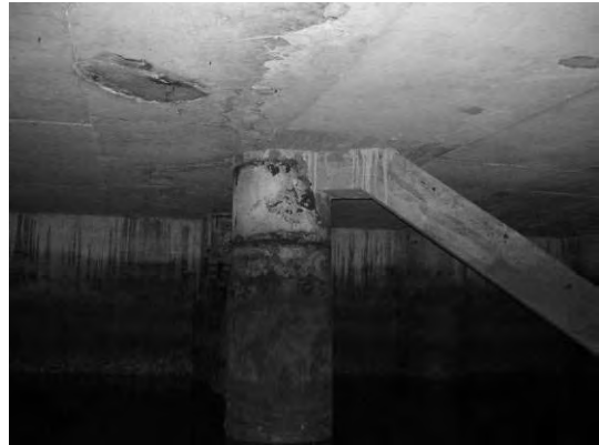
Block 3 Pile 61B
