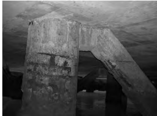
Block 2 Pile 20C-1
