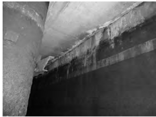
Wall nearby Pile 25C
