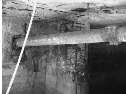
Block 1 Pile 1A and Wall
