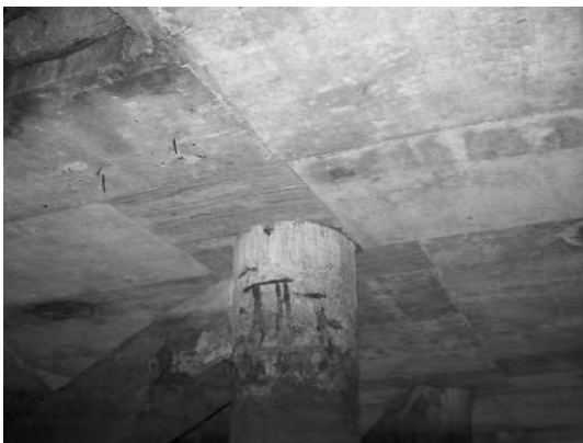
Block 1 Pile 17F-3
