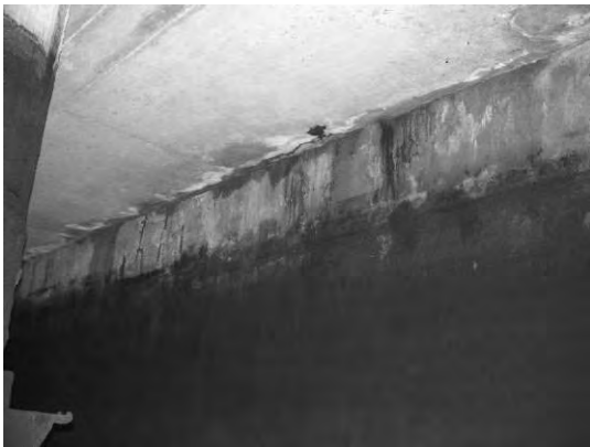
Wall nearby Pile 25C
