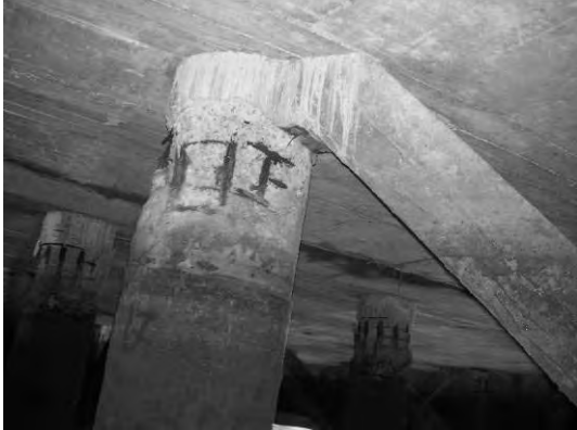
Block 1 Pile 17D-2
