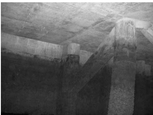
Block 2 Pile 39A ~ 39B
