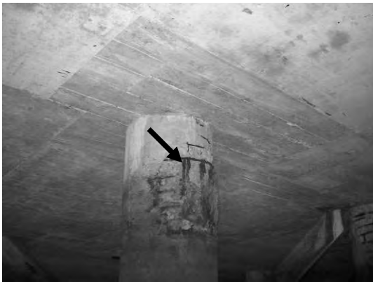
Block 1 Pile 17E-2
