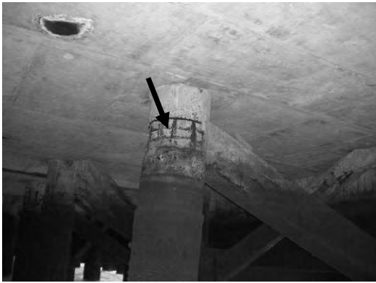
Block 2 Pile 39F
