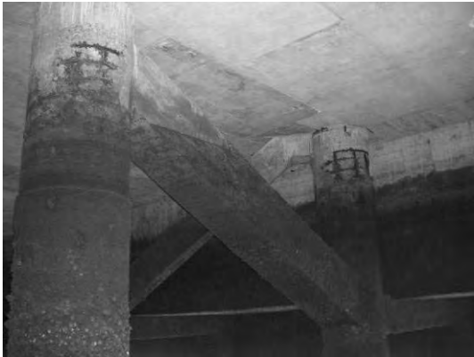
Block 3 Brace bet. Pile 43F & 43G
