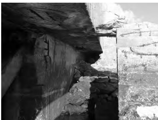
Wall and Slab nearby Pile 1C
