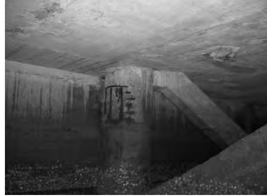
Block 3 Pile 60F ~ 60G-1
