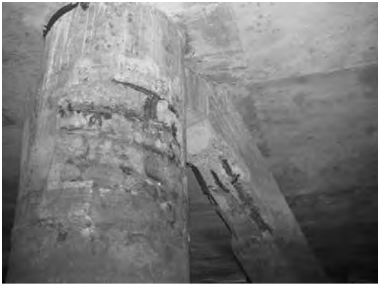
Block 2 Pile 20C-1
