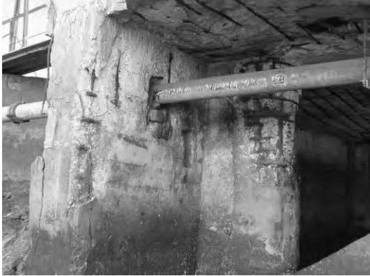
Block 1 Pile 1A and Wall
