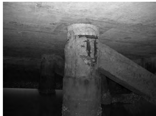
Block 3 Pile 61F
