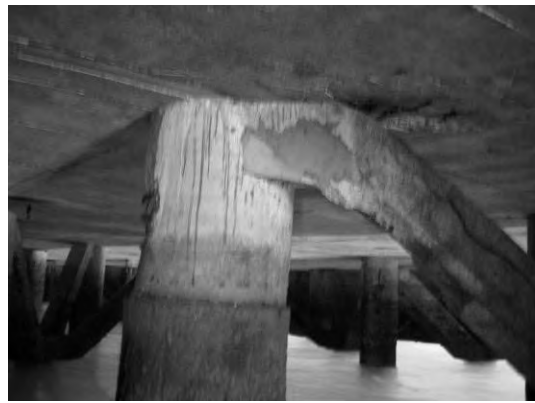
Block 1 Pile 7D
