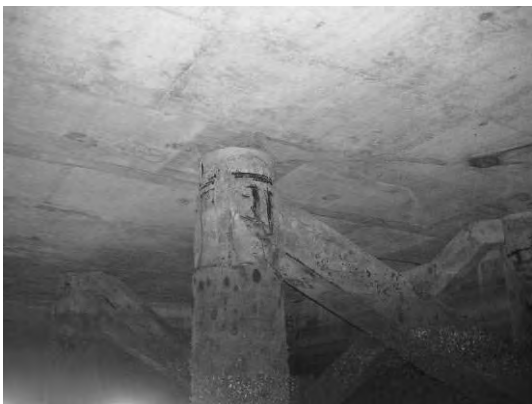
Block 3 Pile 61F
