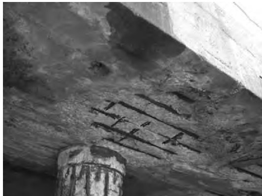
Slab nearby Pile 1B
