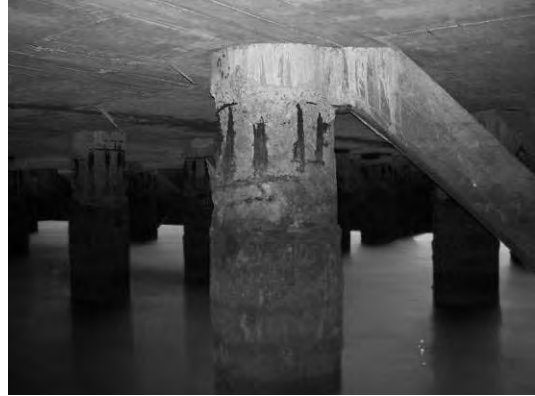
Block 1 Pile 17D-2
