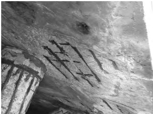
Slab nearby Pile 1B
