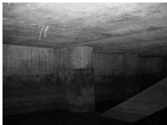
Block 2 Pile 39A ~ 39B
