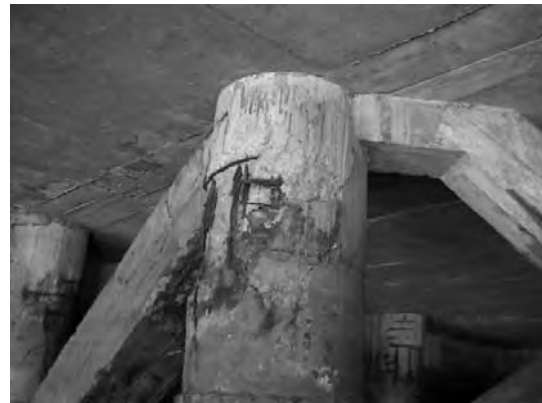
Block 1 Pile 2B-2
