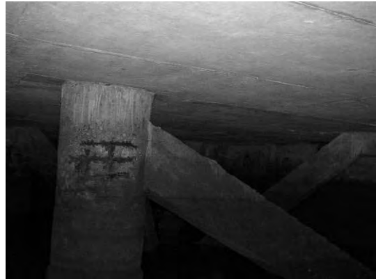
Block 3 Brace bet. Pile 43F & 43G
