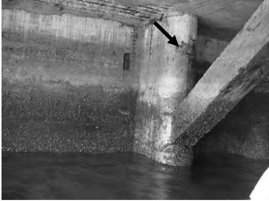
Block 1 Pile 2A
