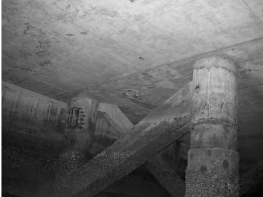
Block 3 Pile 60F ~ 60G-1
