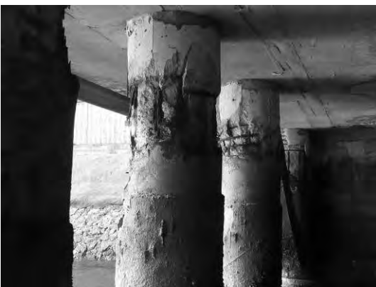
Block 1 Pile 1B & 1a
