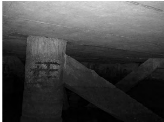
Block 3 Brace bet. Pile 43F & 43G
