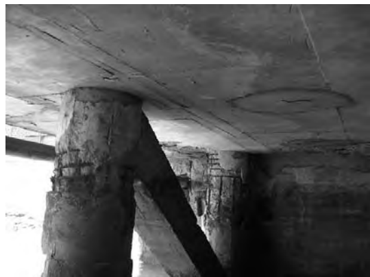
Block 1 Pile 1B & 1a
