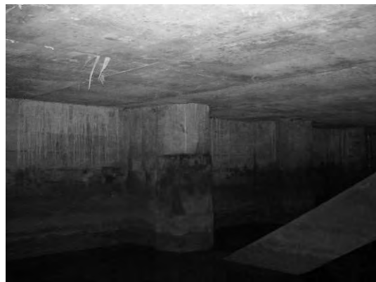
Block 2 Pile 39A ~ 39B
