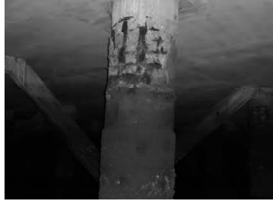
Block 3 Pile 50E-1
