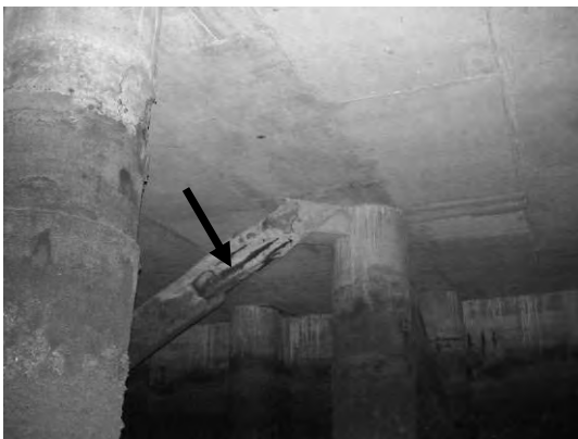
Block 3 Pile 50B
