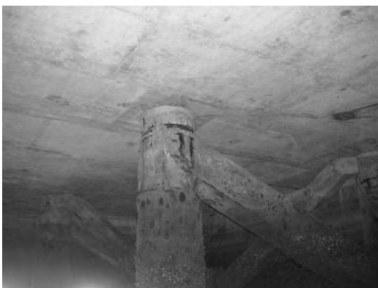
Block 3 Pile 61F
