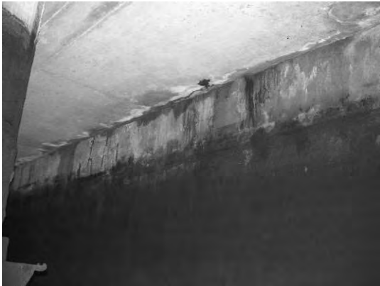
Wall nearby Pile 25C
