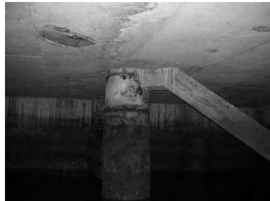
Block 3 Pile 61B
