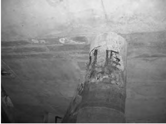
Block 3 Pile 50E-1
