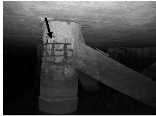
Block 2 Pile 39F
