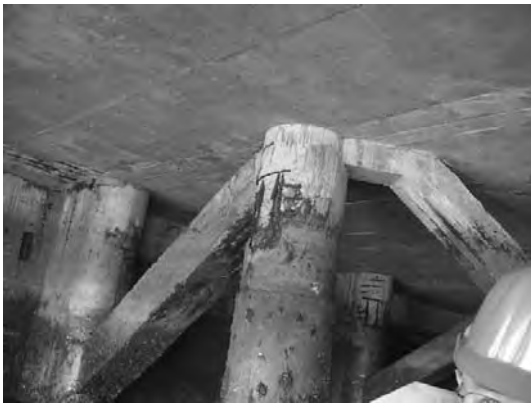
Block 1 Pile 2B-2
