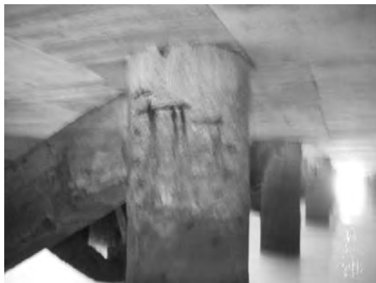
Block 1 Pile 17F-3
