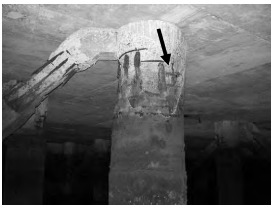
Block 1 Pile 7E-1
