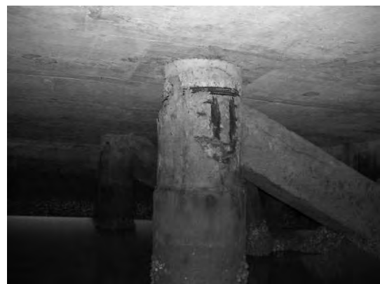
Block 3 Pile 61F
