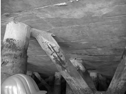
Block 1 Pile 2D-2
