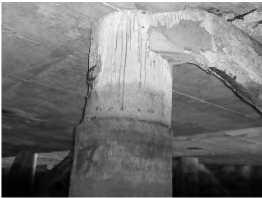
Block 1 Pile 7D
