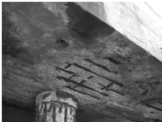
Slab nearby Pile 1B
