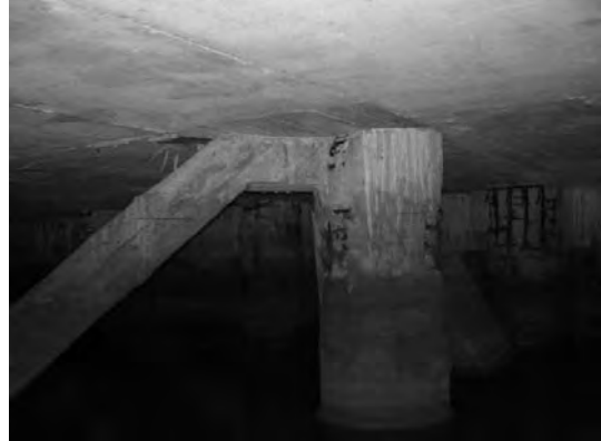
Block 2 Pile 20B
