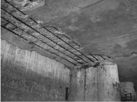
Block 1 Slab bet. Pile 1A& 2A-2
