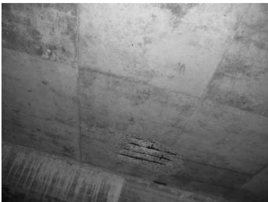
Block 2 Slab bet. Pile 20A & 21A
