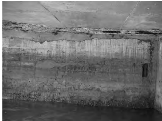
Block 1 Wall bet. Pile 1A & 2A
