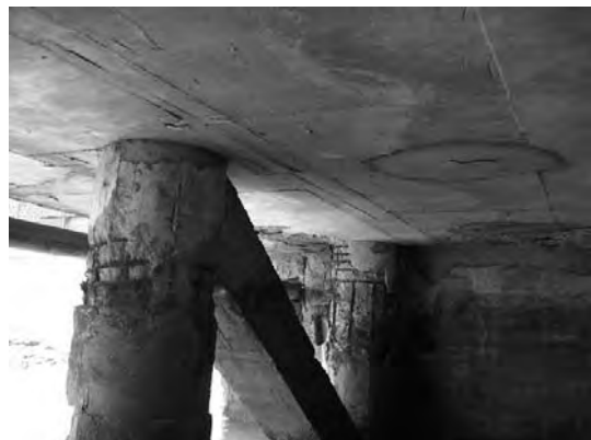
Block 1 Pile 1B & 1a
