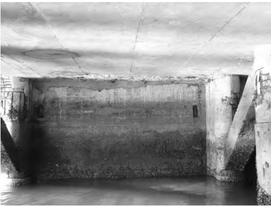
Block 1 Wall bet. Pile 1A & 2A
