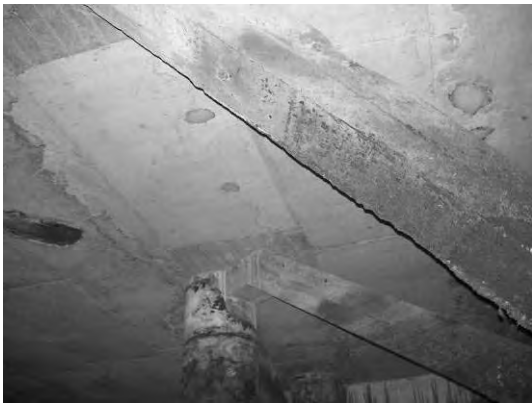
Block 3 Pile 61B
