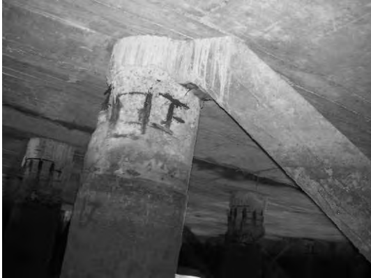
Block 1 Pile 17D-2
