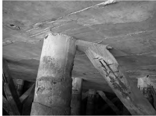
Block 1 Pile 2D-2
