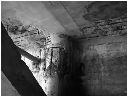
Block 1 Pile 1A
