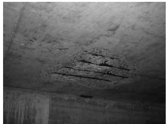
Block 2 Slab bet. Pile 20A & 21A
