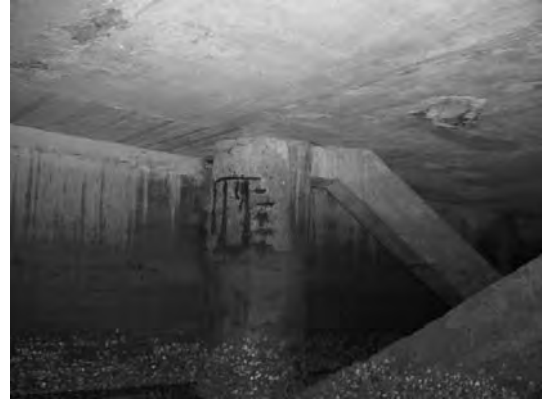
Block 3 Pile 60F ~ 60G-1
