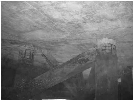
Pile 6B ~ Pile 6C
