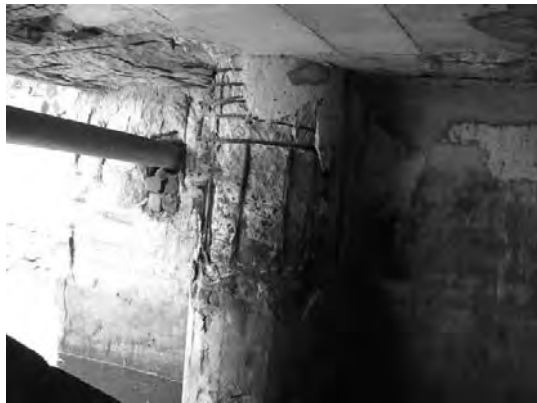
Block 1 Pile 1A
