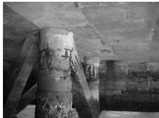
Block 1 Pile 2D-1
