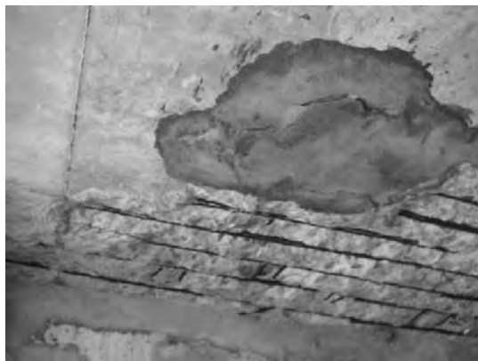
Block 1 Slab bet. Pile 1A& 2A-1
