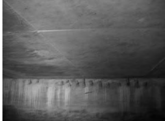
Block 2 Wall bet. Pile 18A & 19A
