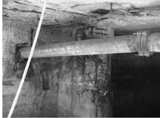
Block 1 Pile 1A and Wall
