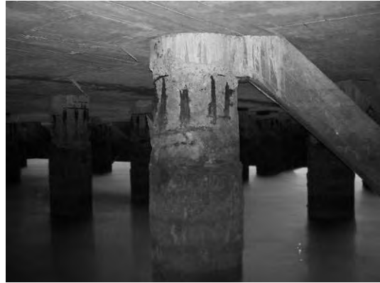
Block 1 Pile 17D-2
