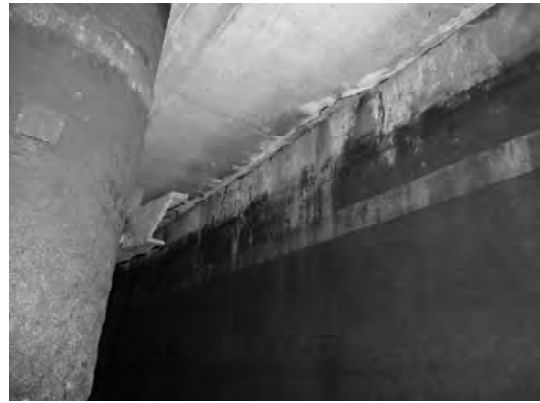
Wall nearby Pile 25C
