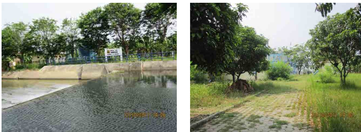
Figure 2.2.6-1 Water Treatment Facility of PDAM
