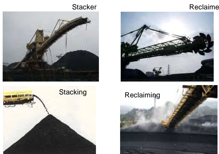
Photo 3.3.3-2 Stacker and Reclaimer
