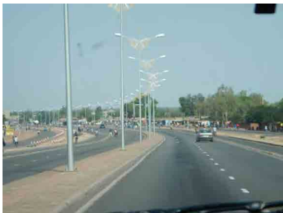
Good road condition surroundings of Ouagadougou
