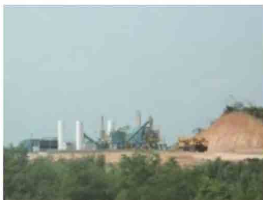
The facility under expansion
