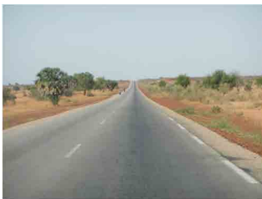
Good road condition
