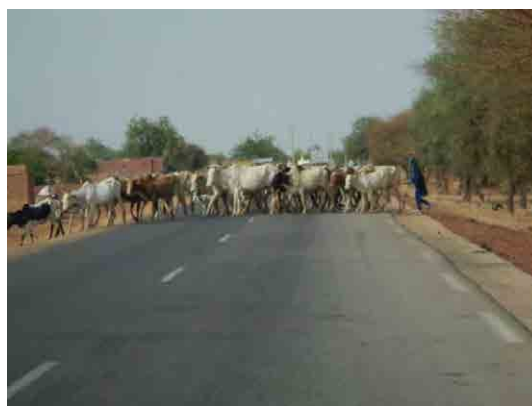
Good road condition
