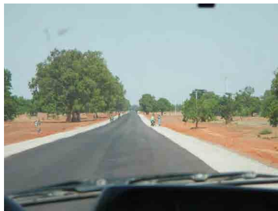
Good road condition near Boromo
