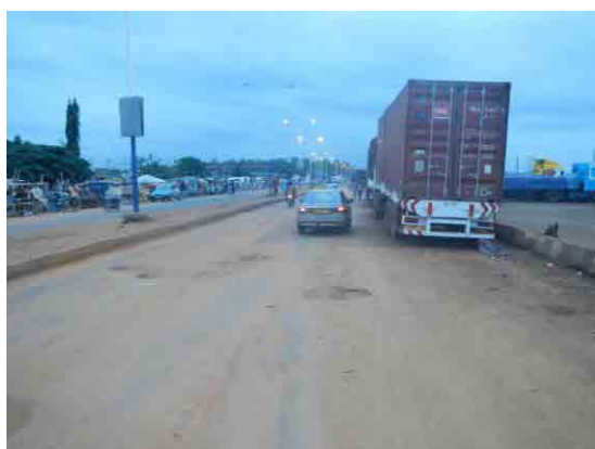
Road condition side of the Sahel terminal
