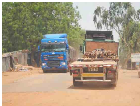
Road Condition in Gaya (2)
