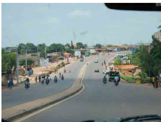
Good road condition In Bobo-Dioulasso
