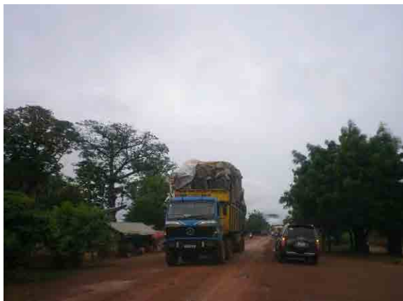
Unpaved section Cinkansé-Dapaong, Togo
