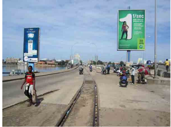
Road-railway combined bridge Cotonou, Benin
