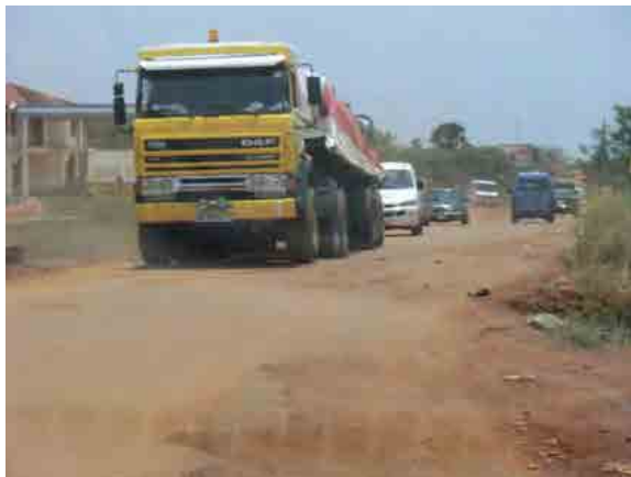
Unpaved section in Coastal Road Near the Togo border, Ghana
