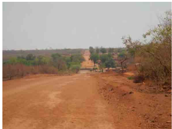
Section under rehabilitation Bella-Gaya, Niger
