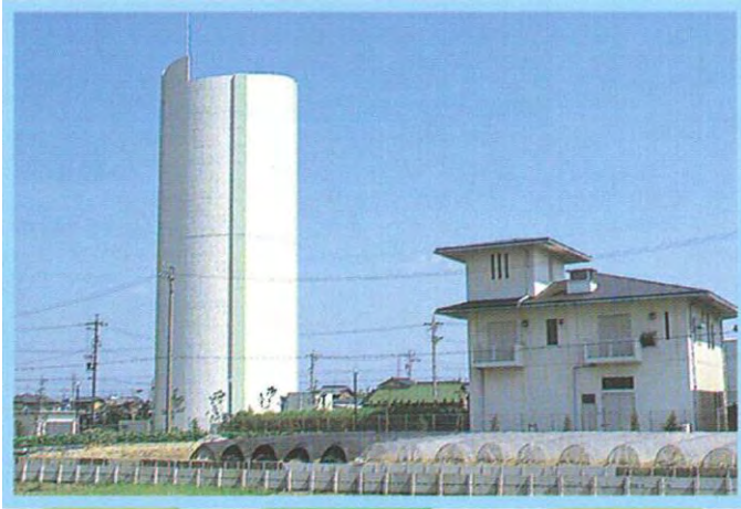
PC tank : 4,000m 3
