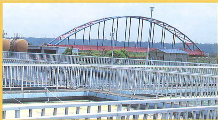
Intake Facility (34,900m 3 /d)
