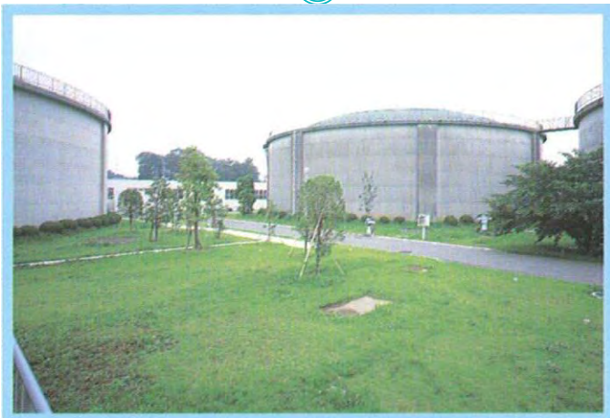
PC tank : 15,000m 3
