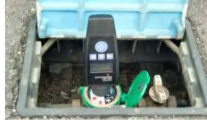
Put LC directly on water meter and push the button
