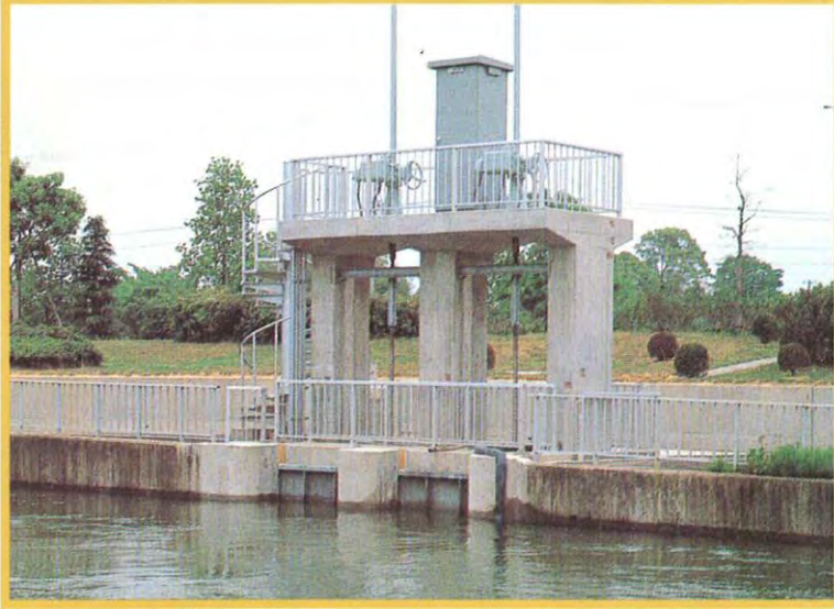
Intake Facility (290,000m 3 /d)
