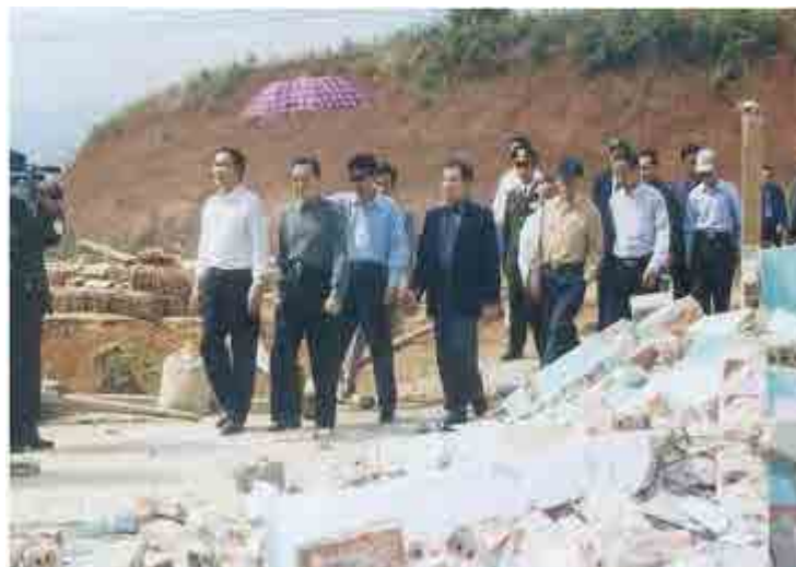
Figure 4.2.2-3 A collapsed masonry structure by Dien Bien Phu (DBP) earthquake on 19 February 2001 (Source : The seminar document by IBST)
