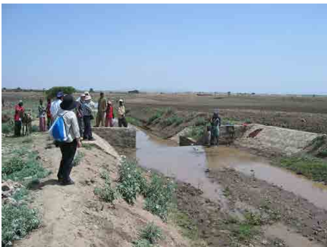
ドドタシレ Spate Irrigation Scheme (幹線水路)
