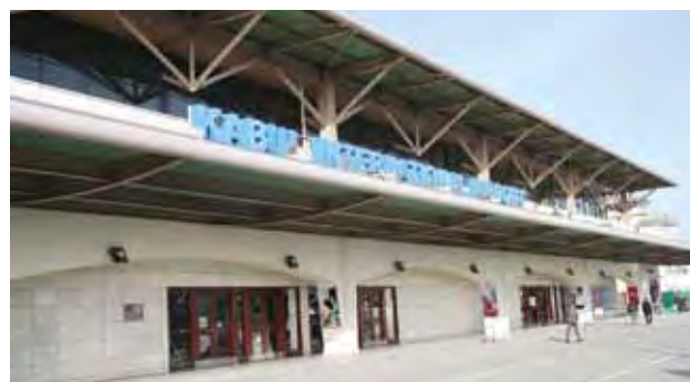
Grant Aid was provided for the construction of the international airport terminal in Kabul, the capital of Afghanistan. The airport is now functioning as a valuable link between Afghanistan and the world with a large increase of passengers from 300,000 before the project to more than 900,000 at present. (Photo by Sayad Jan Sabawoon)
