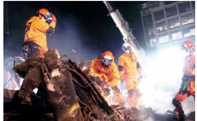
Rescue Team members conducting rescue activities
