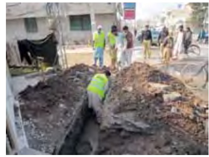
A water pipe is repaired in the Pakistan city of Lahore
