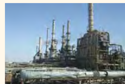
The Basrah Oil Refinery
