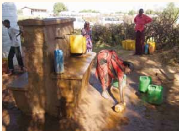
A water supply facility in Gode in the Somali region of Ethiopia
