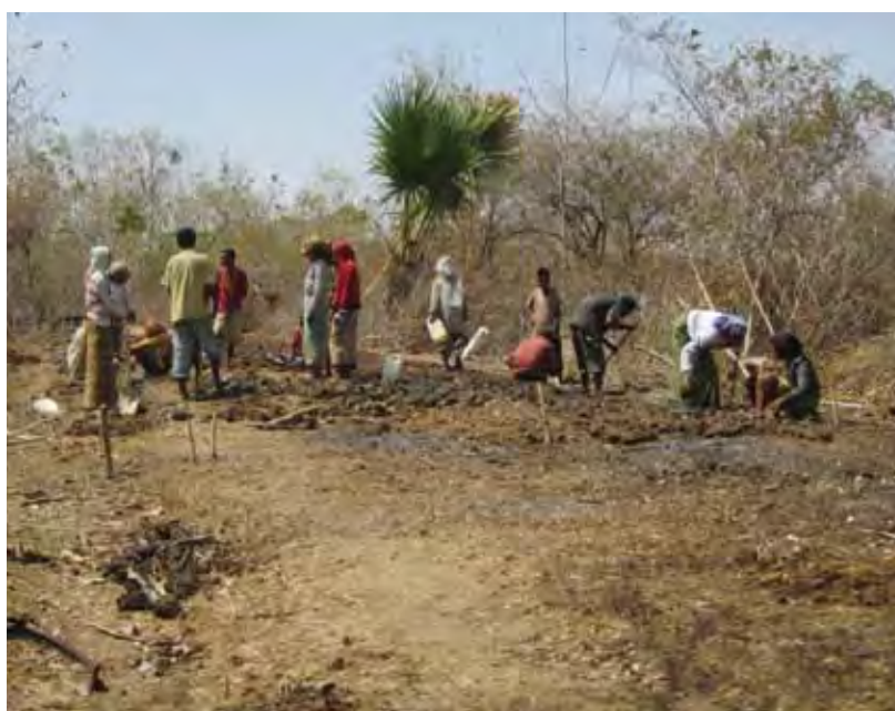
Local residents help build community roads (Timor-Leste)
