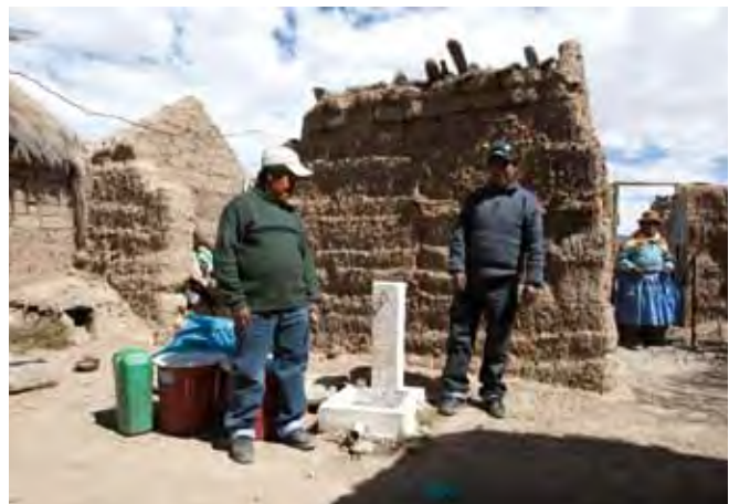
Pipes link the water storage tank with houses in the community (Bolivia: “Water is Health and Life” Project)
