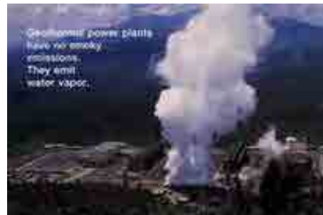
Typical Geothermal Power Plant
