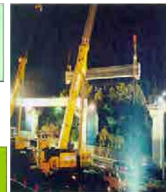
Construct Work at Night
