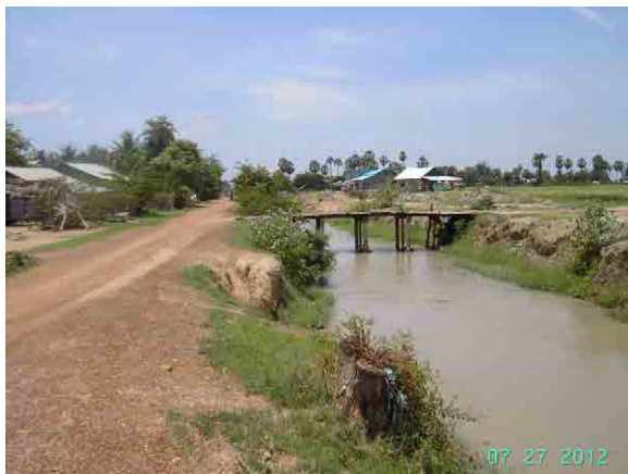
Existing south main canal
