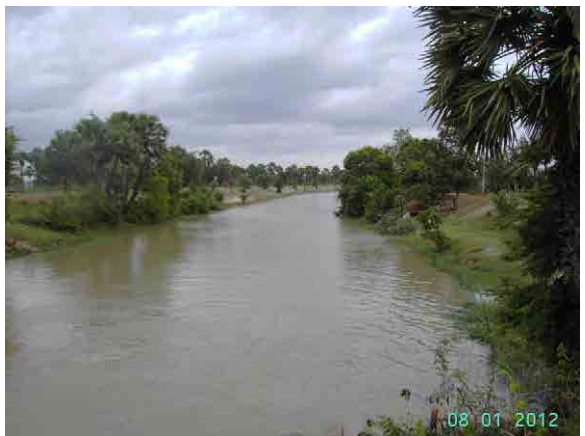
Existing north main canal
