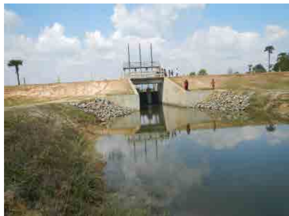
Intake of Khpob Krous Reservoir
