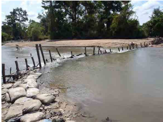
Temporary Weir for Daun Pue Intake made with Sand Bags and Wooden Material
