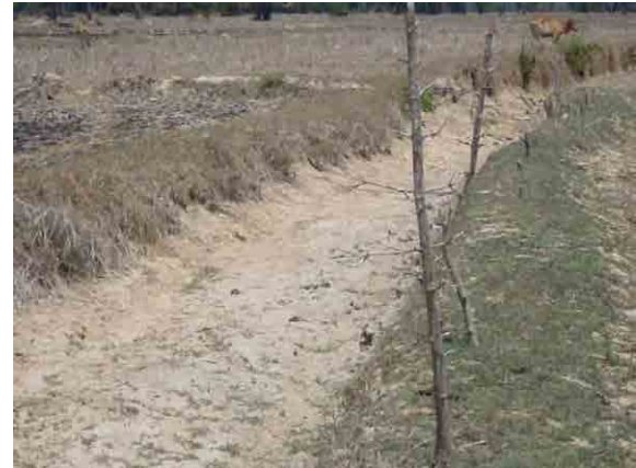
Existing Secondary Canal
