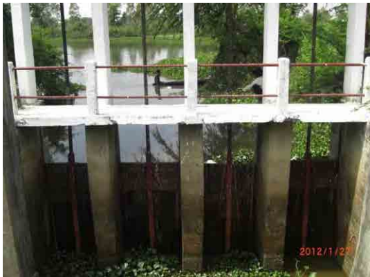
Spillway of Lake Tonle Bati (Downstream)
