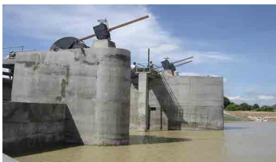
Rehabilitated Mechanical Spillway Gates
