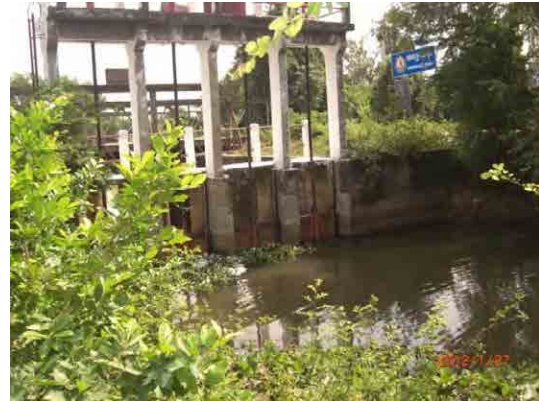
Spillway of Lake Tonle Bati (Upstream)
