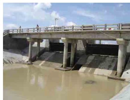
Downstream View of Spillway Gates
