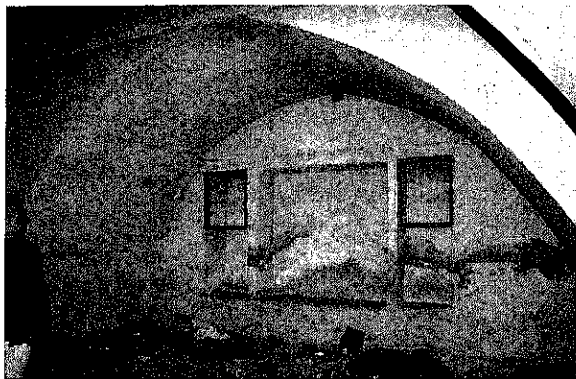
Barrel Vault Ceiling
