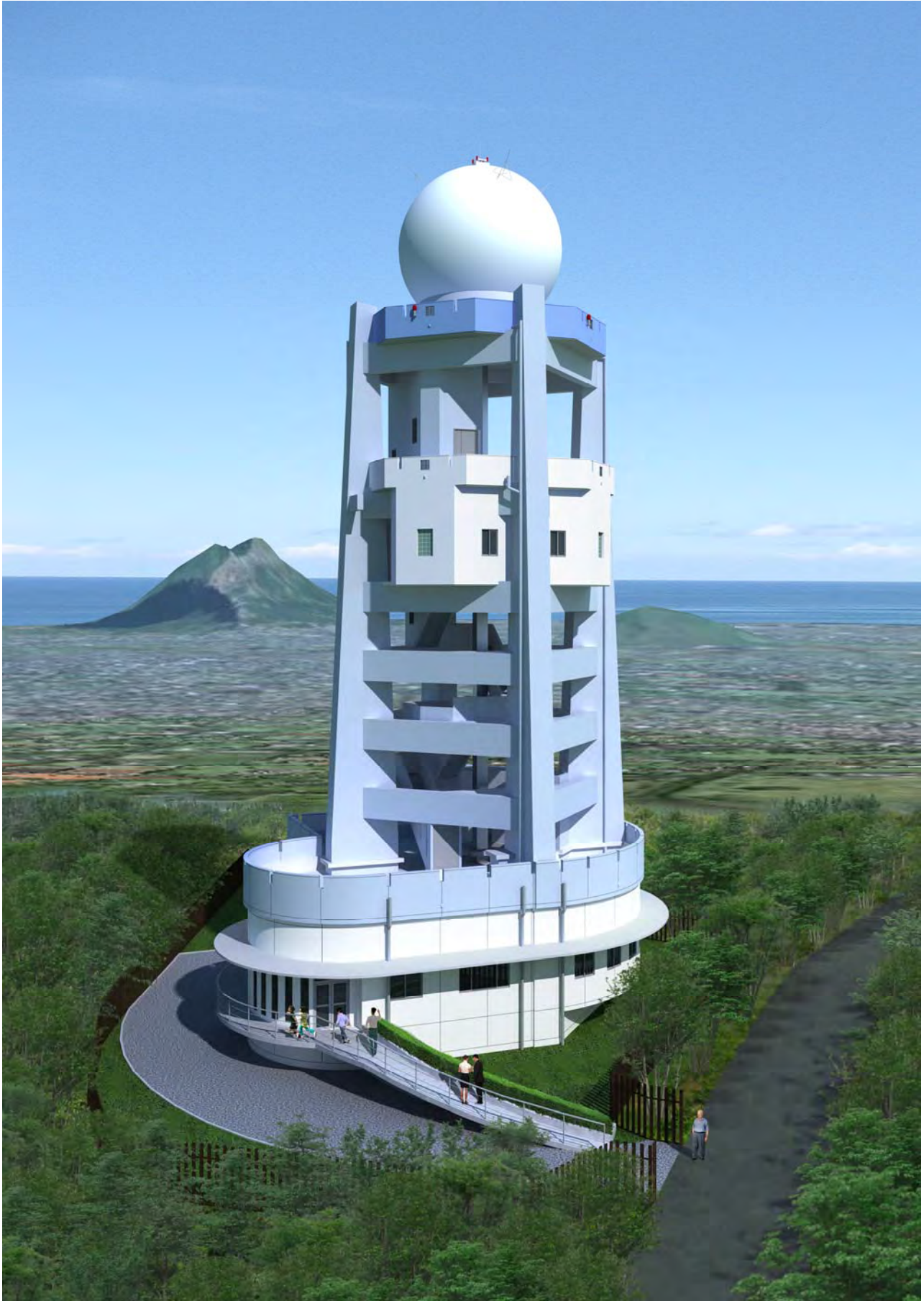
Trou-aux-cerfs Meteorological Radar Tower Building
