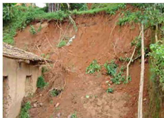
Photo 5 Landslide in Rwanda;
