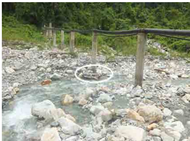
Figure 5.2.10 Aqueduct in Gelephu (Sarpang) Tarulay Irrigation Area
