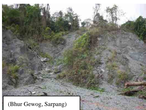
Figure 3.1.20 Eroded Fracture Zone in Lesser Himalayan Belt
