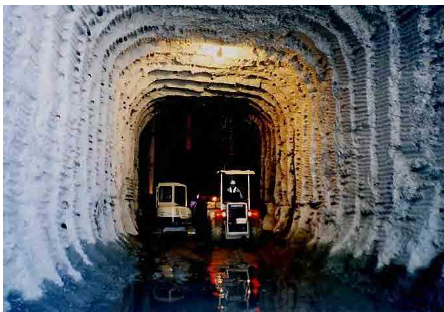
Photo 6.2.1 Inside View of Dam Piercing (Okutadami Dam)
