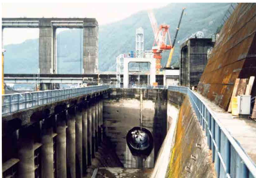
Photo 6.2.2 Front View of Dam Piercing (Akiha Dam)
