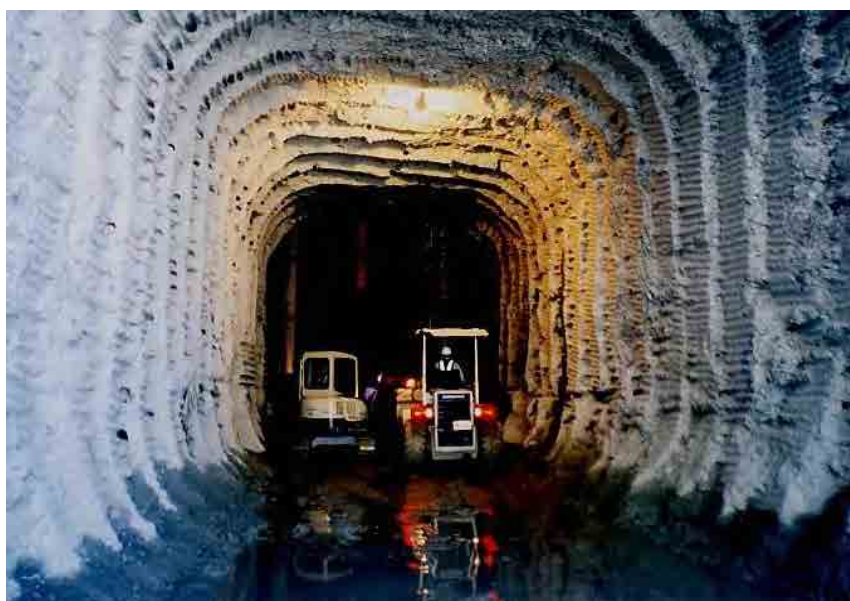
Photo 6.2.1 Inside View of Dam Piercing (Okutadami Dam)
