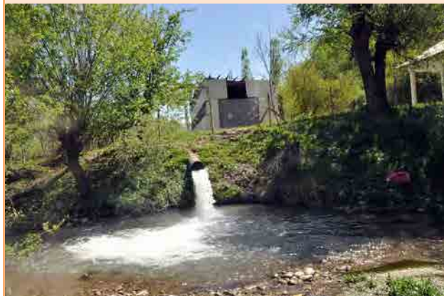
UNDP Pump Station
