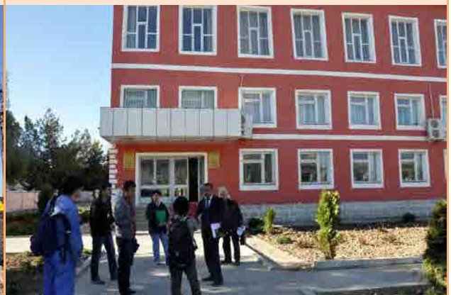
Muminobod Administration Office
