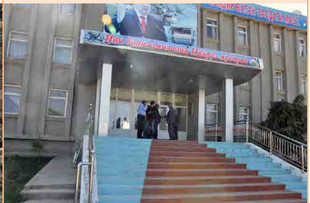
Khovaling Administration Office
