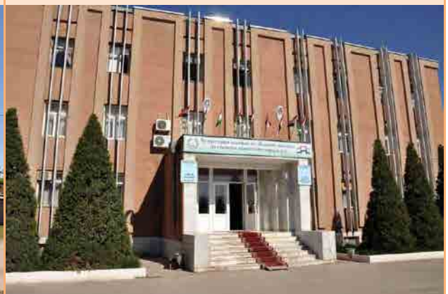
Bohtar Administration Office
