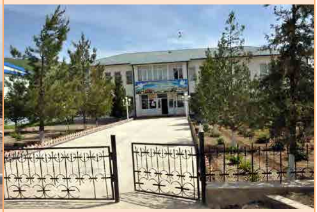
Baljuvon Administration Office
