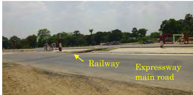
Railway crosses expressway. Road traffic blocked with manually operated gate
