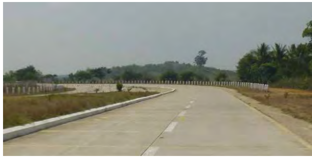
Entrances to curves give the impression of being too sharp
