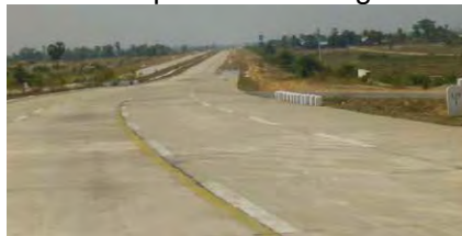
⇒ Road widens to four lanes between off- and on-ramp
