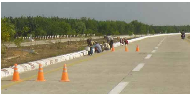
Painting curbstone along the median. Traffic regulations are extremely rudimentary
