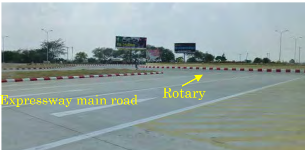
In suburban Mandalay, traffic slows due to rotary-style on/off ramps (speed limit 60kmh on main expressway road)
