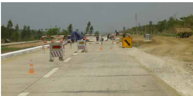
Both two lanes closed. Vehicles directed to detour on unpaved part
