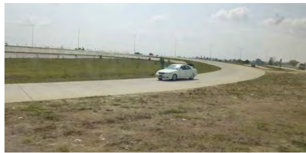
Some interchange ramps have no safety facilities whatsoever Nay Pyi Taw interchange ramp (extremely poor visibility)
