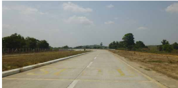
Zones with sharp curves have a speed limit of 80km/h "SLOW" warning sign painted on road surface
