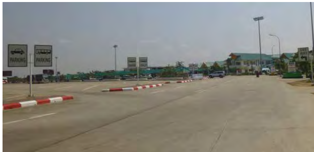
Rest facility with a restaurant (Rest Camp)
