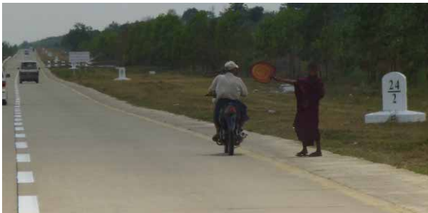
Expressway is not completely closed off, meaning that vehicles and people may enter or cross at locations other than inter changes.
