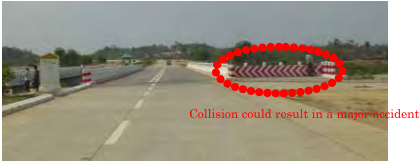
Bridge area with high risk of collision
