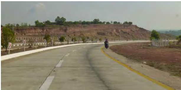
In sharply curving sections, there are arrow signs installed (Motorcycle is going the wrong direction)
