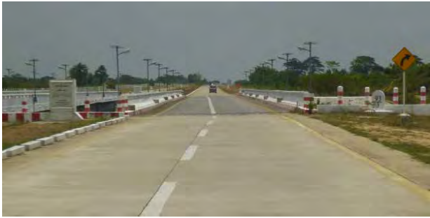
Abrupt a alignment of carriageway
