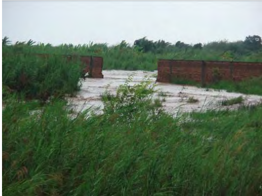
Flow of Nthahangwa River during 2009 flood event broke several brick wall of Port Bujumbura.
