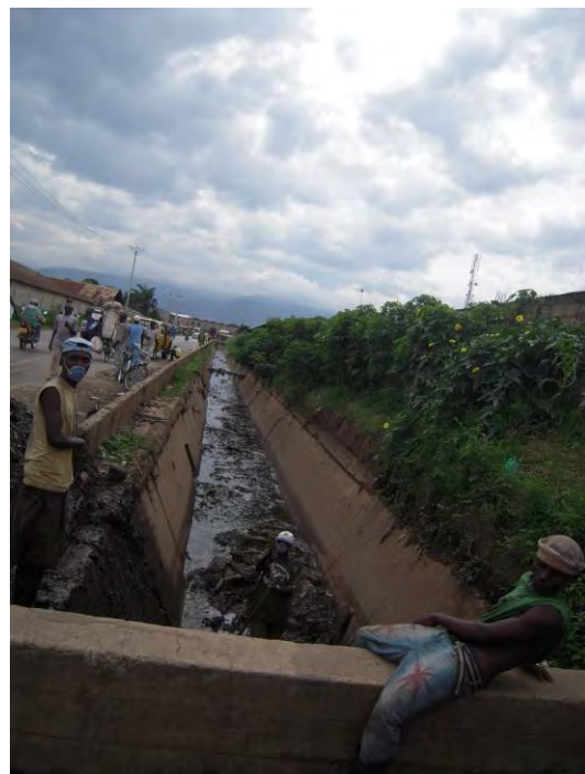
Clean-up work of Buyenzi Channel (Photo taken on March 2012)
