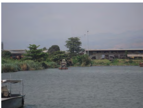
Overview of Existing Port around Outlet of Buyenzi Canal (Photo taken in Sep. 2011)
