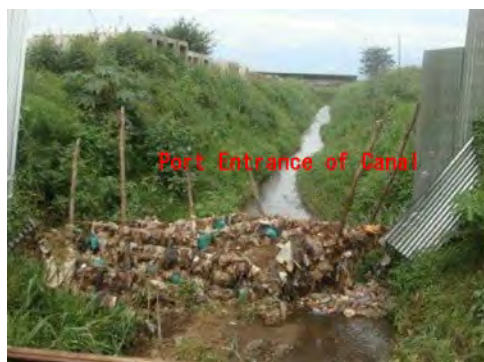
Photo 11.1: Canal Out of Port Fence
