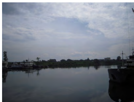
North-Side Overview of Existing Port (Photo taken in April 2012)
