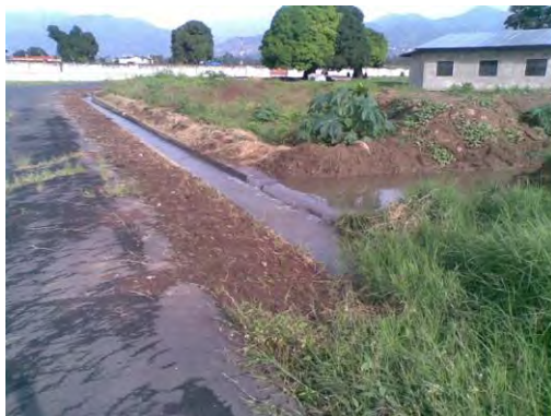
Drained water from removed sludge run down to a nearby channel without any treatment, then eventually back to port.
