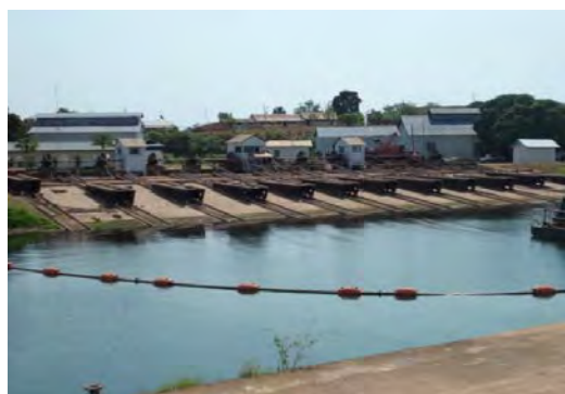
Photo 3.23: 11 Horizontal Cradles of Kigoma Slipway
