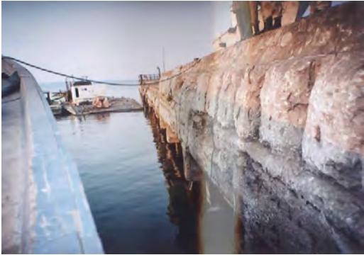
Photo 3.21: Damaged Concrete Deck and Piles at Kalemie Port
