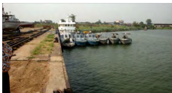
Quay-wall: Gravity type Bollard: 25 tons
