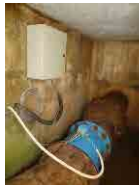
Unused electromagnetic flow meter
