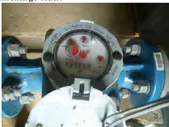
Flow meter in underwater pump
