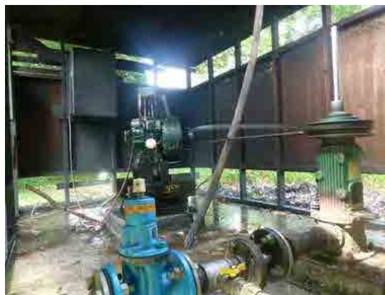
Diesel engine pump
