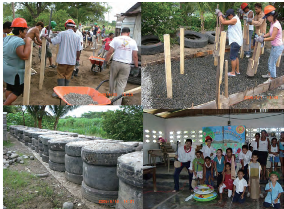
Figure 7: Construction of Used-tire Dyke in Costa Rica
