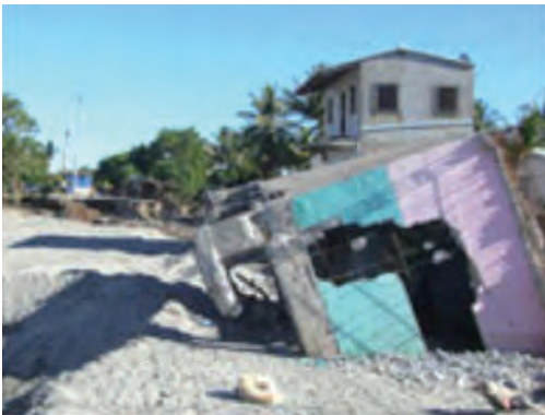
(Above) House destroyed by Hurricane Ida in Las Ojas community in November 2009
