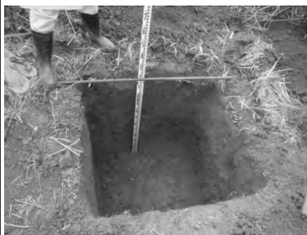
GL to 1.15m: Top soil of clay. Deeper than 1.15m: Manual excavation is rather difficult due to rather large grain diameter of hard laterite. Long-term allowable bearing capacity: Over 5t/m 2
