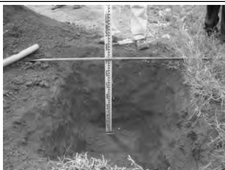
GL to 0.70m: Top soil of clay with small particle of hard laterite. Deeper than 0.70m: Difficult to excavate manually due to hard laterite. Long-term allowable bearing capacity: Over 10t/m 2
