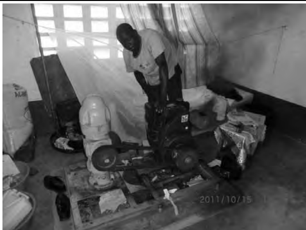
Broken engine and pump for the existing piped water supply system. A pump operator stays in the pump house. (Awere RGC)
