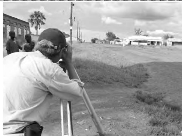
Topographic survey (Corner Kilak RGC)
