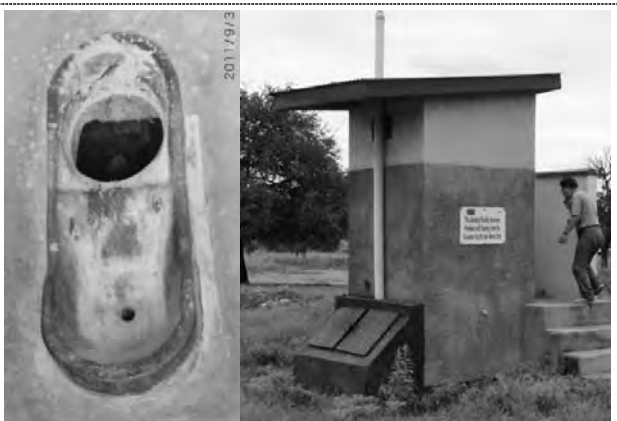
Existing ecosan toilet - Solid and liquid wastes are collected separately. (Agago RGC)
