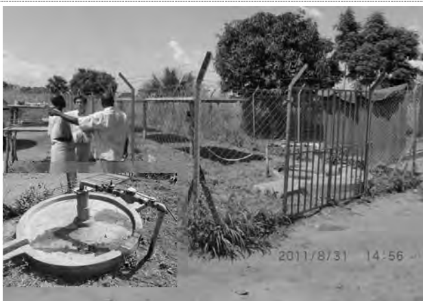
Existing piped water supply system operated with solar power generation utilizing a borehole facility for hand pump. (Kitgum Matidi RGC)
