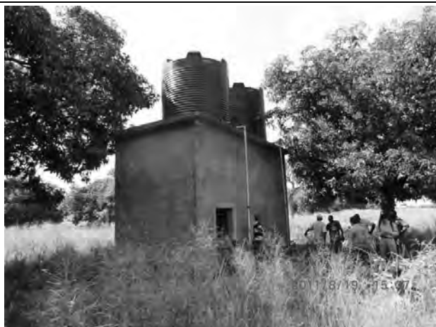
Abandoned pump house for piped water supply system. Domestic animals are fed in the house. (Corner Kilak RGC)
