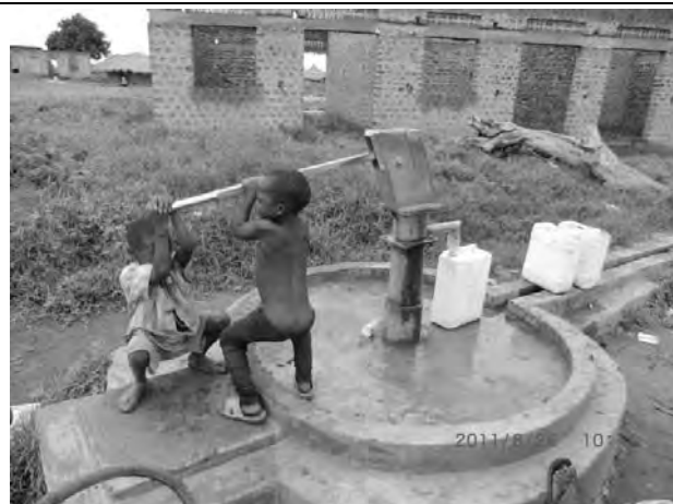
Existing borehole with hand pump - handle operation is rather hard for children due to low water level. (Kochi Goma RGC)
