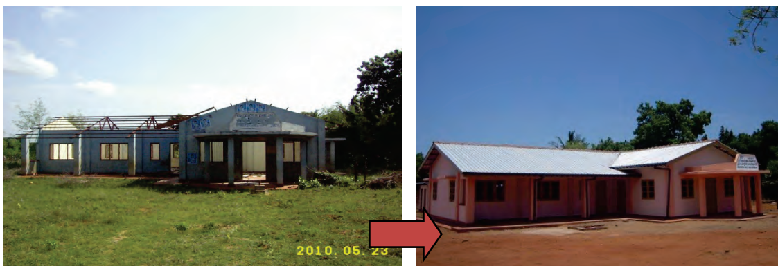
Damaged multi-purpose hall in Ganeshapuram Reconstructed multi-purpose hall in Ganeshapuram
