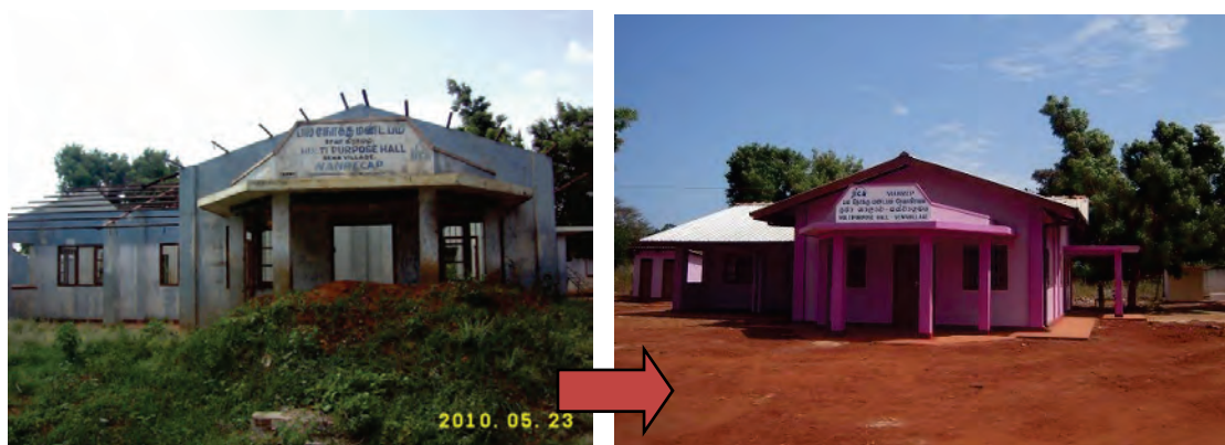
Damaged multi-purpose hall in Sewa Village
