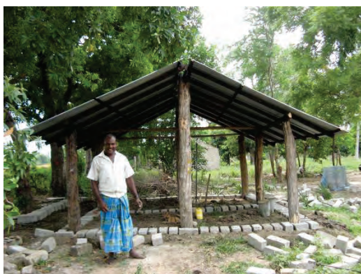
Building a temporary house (C K Adampan)
