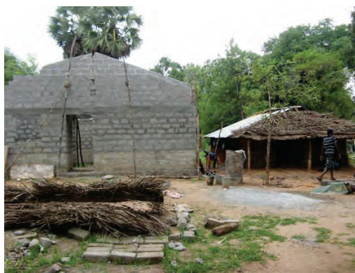
A New House is under Construction (Vilathikulam)
