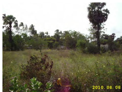
Pre-school building in Periyakulam was completely damaged
