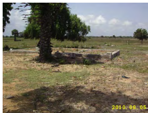
Damaged Pre-school building in Vellankulam
