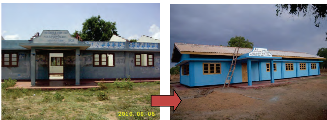
Damaged multi-purpose hall in Pali Aru Re-constructed multi-purpose hall in Pali Aru
