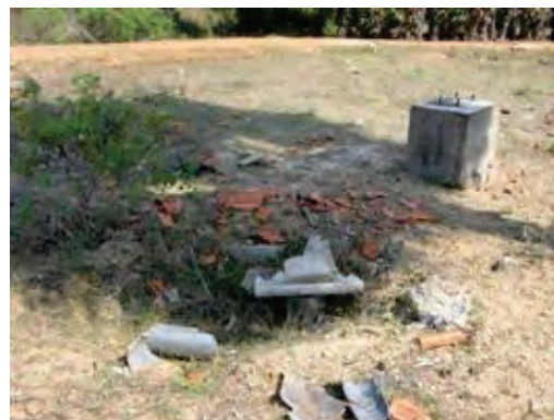
Destroyed tube well
