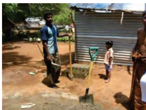
Cement block making
