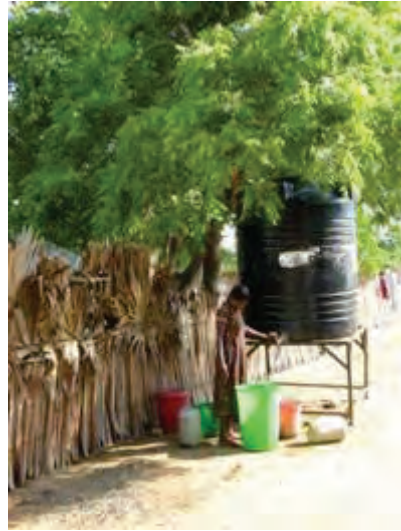
water supply by ZOA
