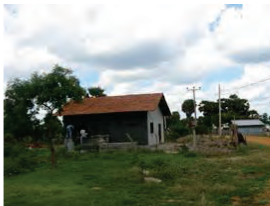
Permanent houses are under re-construction
