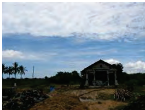
A church under reconstruction
