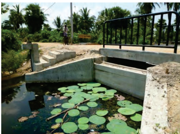
Irrigation Tank Spillway at Periyakulam, Parapankandal GN Division
