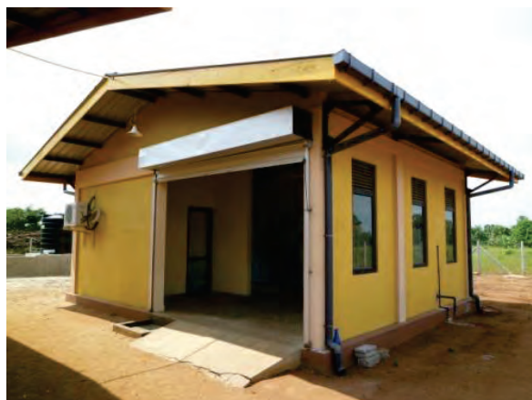
Poultry Hatchery Building at the Breeding Farm in Cheddiyarmagan Kaddaiadampan GN Division
