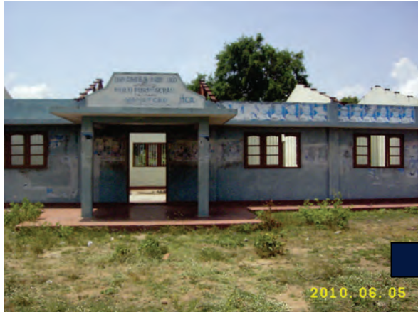
Multi-purpose Hall at Pali Aru, Pali Aru GN Division before the rehabilitation by community contract
