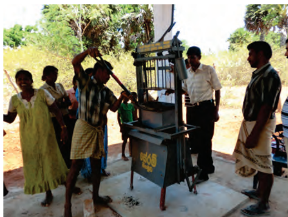
Cement block making at Ganeshapuram, Vellankulam GN Division
