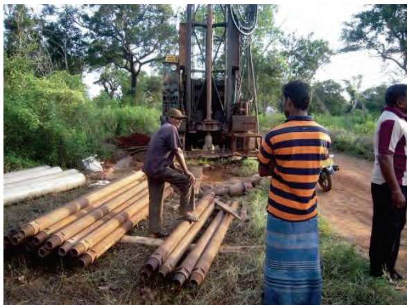
Drilling of Tube Well at Sinna Valayankaddu, Parasankulam GN Division
