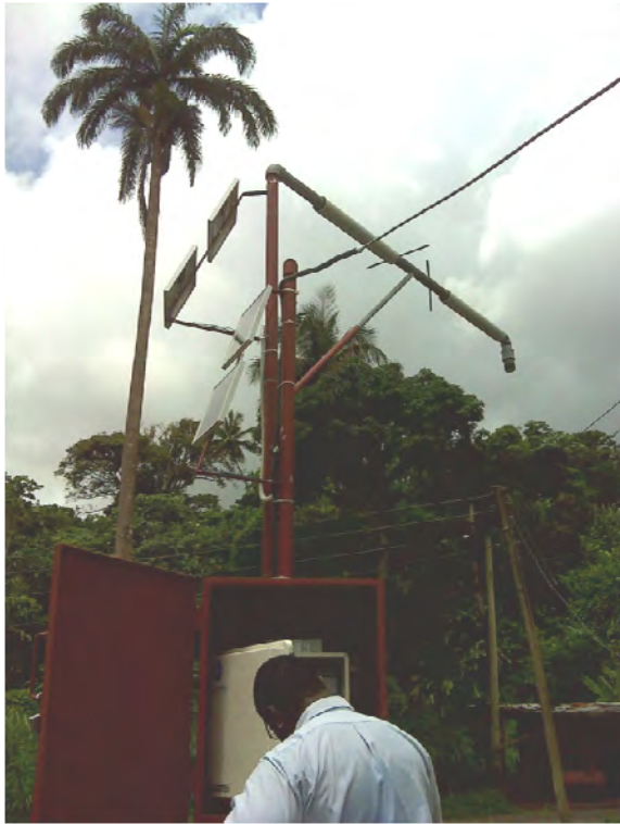
New Water-level Station (Grenada)
