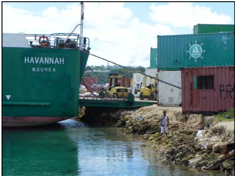
Photo-7 Northern Revetment used for ro-ro ships
