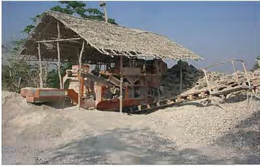
Photo-2-2-9 A quarry (crusher made in Japan)
