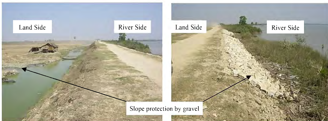
Photo-2-2-11 Reinforcement of embankment with gravel materials
