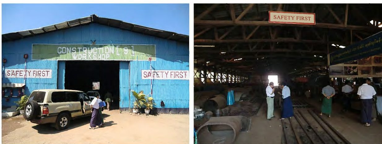
Photo-2-2-4 The workshop and the warehouse for spare parts of Con (9)
