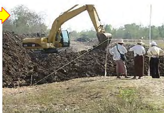
Temporary Placing (left side of back-hoe)
