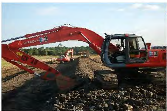
Slope finishing work by back-hoe
