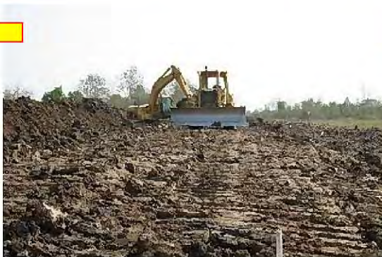
Stripping, leveling and compacting of polder embankment works by bulldozer
