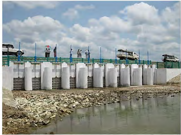
【Restored sluice (Pilot Project)】
