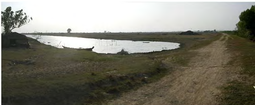
Photo-2-2-8 Enclosed site of tributary flow near Danechaung Water gate
