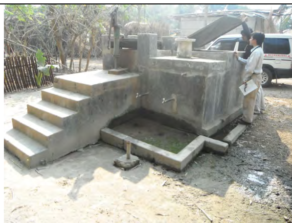
Photo-4 : Existing Arsenic Iron Removal Plant (AIRP) (Bergobindapur village, Jessore)
