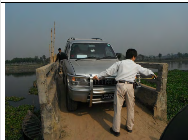
Photo-9 : Narrow bridge (Bergobindapur village, Jessore)
