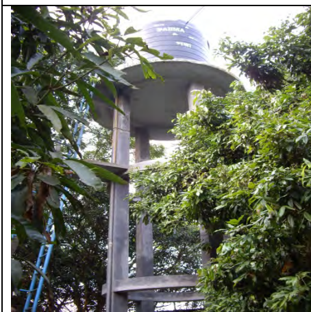
Photo-3 : Water storage tank of existing piped water supply facility (Pabna)
