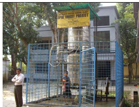
Photo-2 : Groundwater Arsenic Removal Plant by project of DPHE-UNICEF (Pabna)
