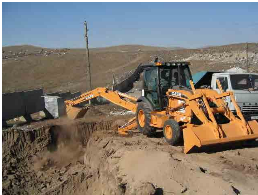
Figure 1: Wheel type loader with Excavator
