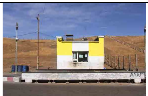
Side view of truck scale and control house
