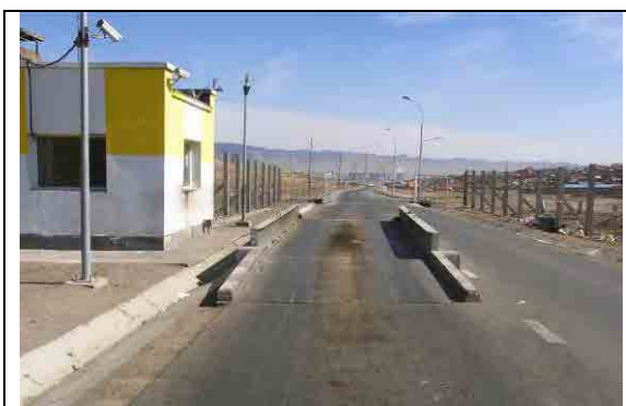
View of entrance looking out of the disposal site
