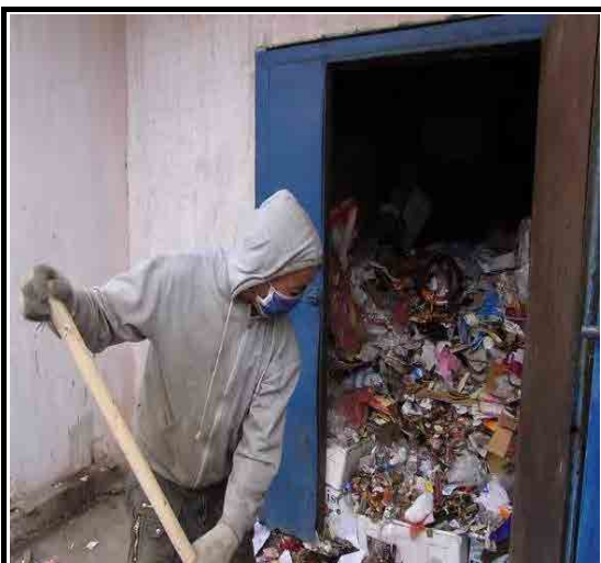
Waste collection before closure of dust chute in SBD-7: Wastes were not in the bags and accumulated inside. Collection worker needed to scrape out the waste and load on the vehicle.
