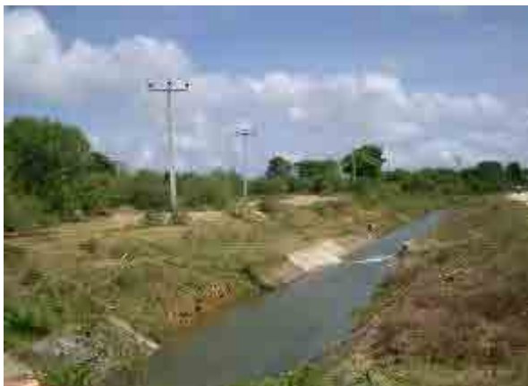
支線土水路の侵食 (Branch Canal-2, Mayurapura Block)
