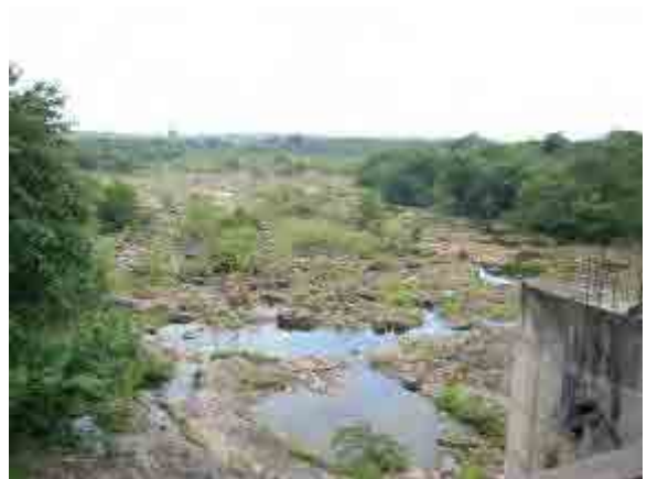
ダムの放流路 (Low Bank Main Channel from Uda Walawe Tank)
