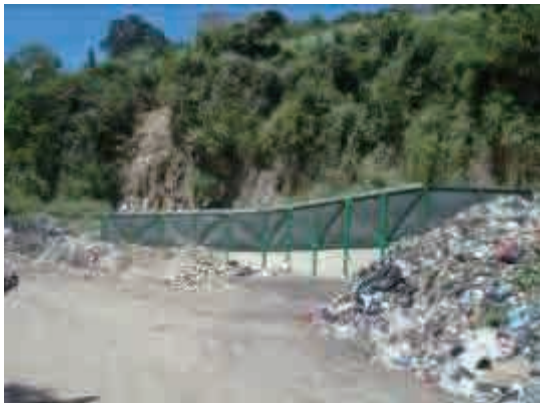
Aragon transfer station
