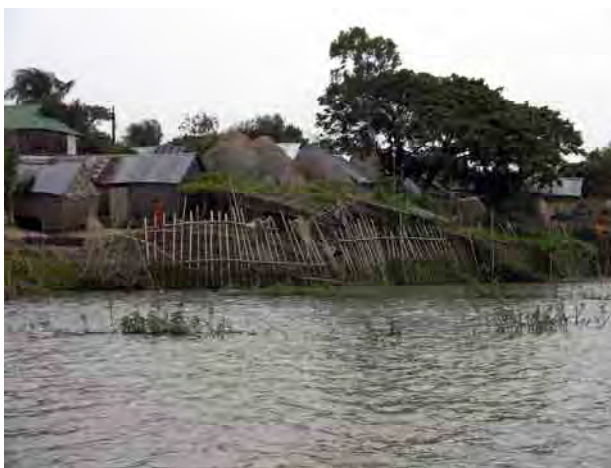
Revetment works provided by the people using bamboo and grass to protect their mound from wave action and erosion in haors (Khaliajuri, Netrokona)
