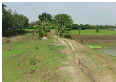
3a. Full Flood 堤防
