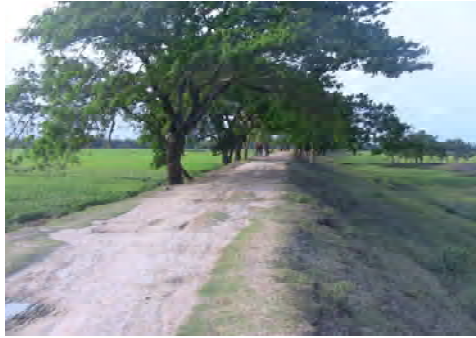
1a. Full Flood 堤防 (1)
